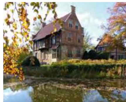
Haus Bisping, Drensteinfurt
